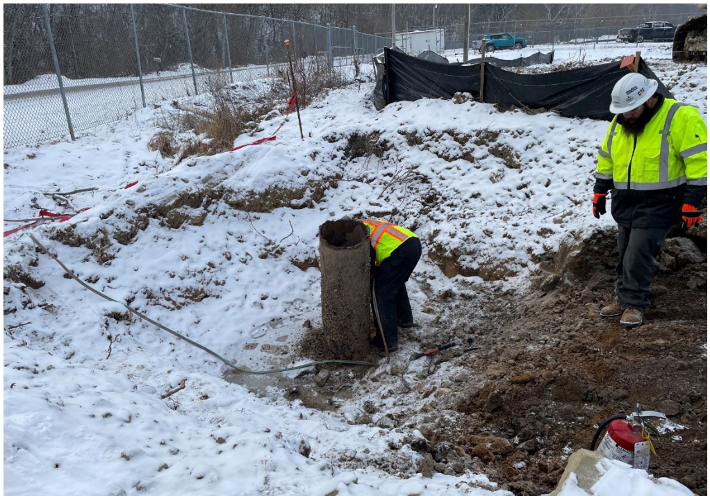
PHOTO 7: Cutting surface casing below new ground elevation.
