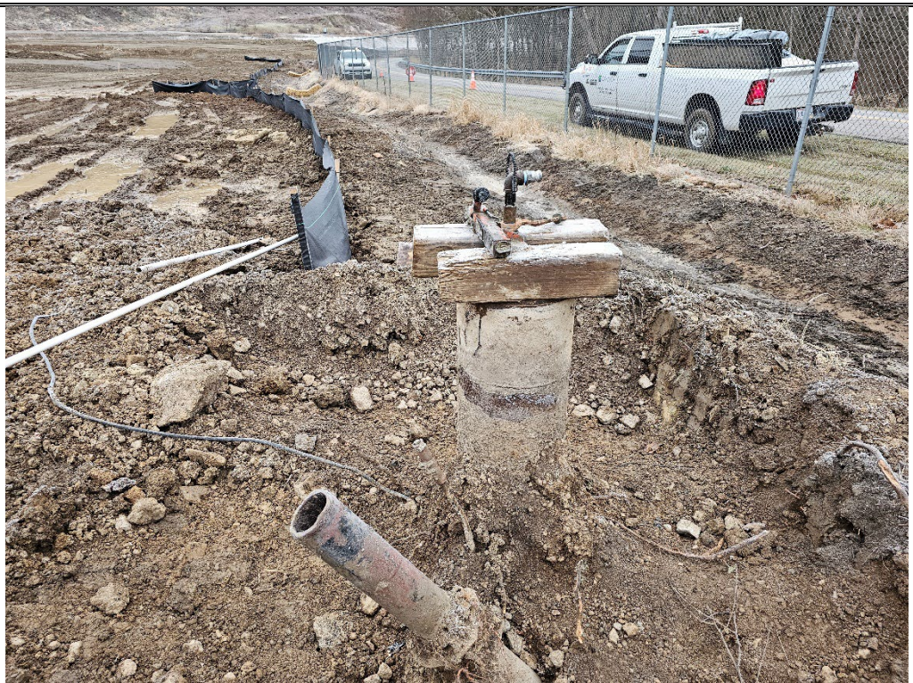
PHOTO 4: Tremie pipe staged on top of well casing.
