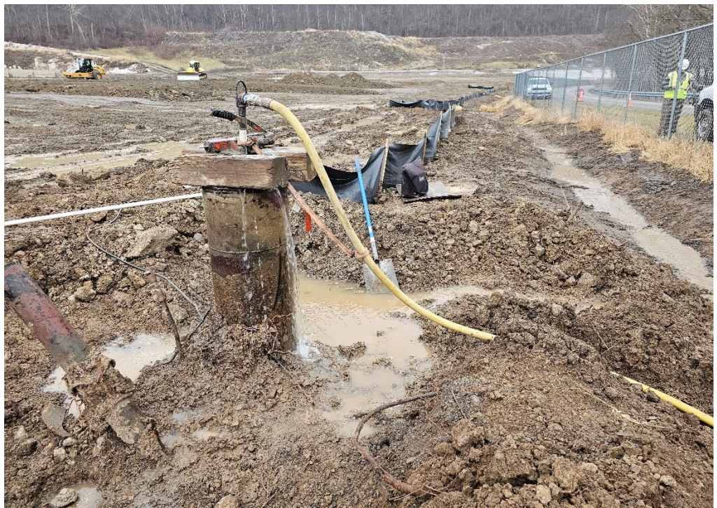
PHOTO 3: Static water was removed from the well.
