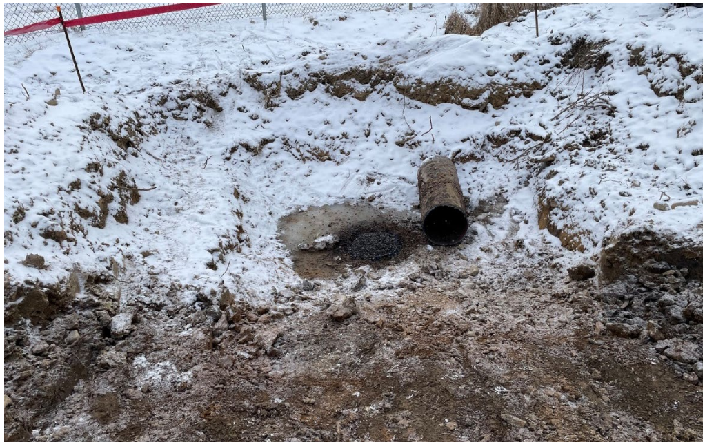
PHOTO 8: Final sealing of remaining casing with hydrated Hole Plug®.
