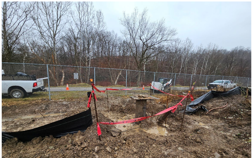
PHOTO 6: T-posts wrapped in caution tape surround the well after grouting.
