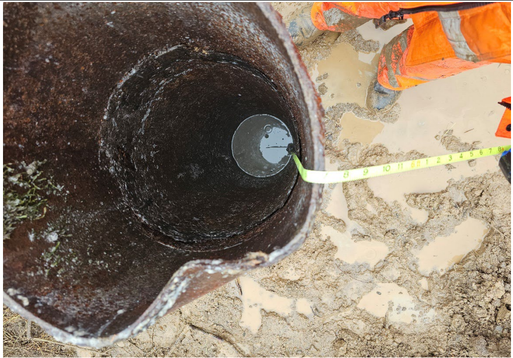
PHOTO 5: The well was grouted 3ft below grade.
