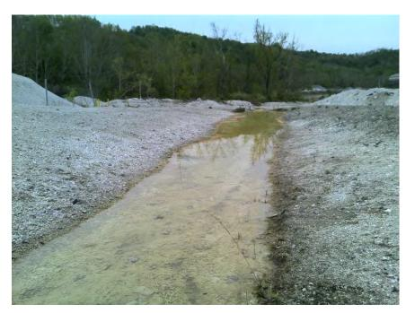
**Feature:** Tributary LL **Date:** 5/11/2018 **Description:** Tributary LL is a constructed drainage designed to discharge stormwater into Cross Creek through a series of culverts.
