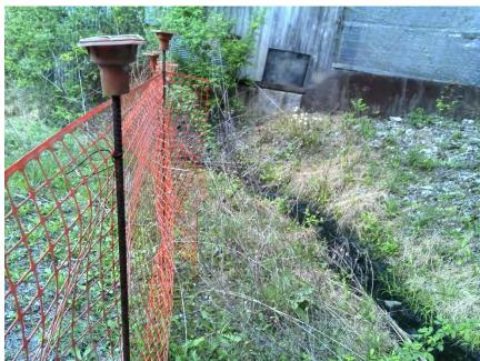
**Feature:** Tributary OO **Date:** 5/9/2018 **Description:** Tributary OO has developed as the result of trenching near a blocked pipe located alongside the south mill. Flows from this drainage are captured in a ponding area that does not demonstrate wetland characteristics.
